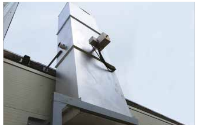
Creation of a soundproofed ducting chimney
