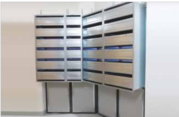
Acoustic reclamation of doors in hydroelectric power plants through the application of silencers with baffles
