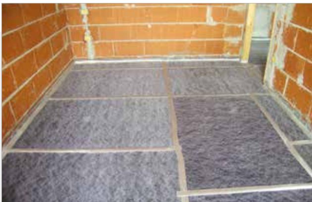
Floor acoustic insulation
