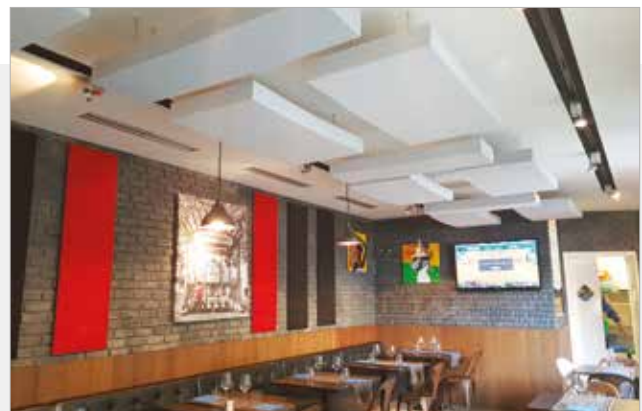
Acoustic correction inside a restaurant
