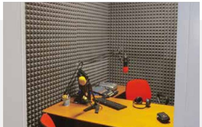
Insulation in a radio recording studio
