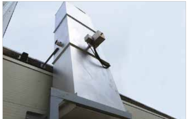
Creation of a soundproofed ducting chimney
