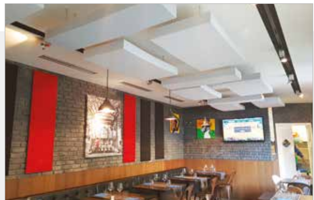
Acoustic correction inside a restaurant
