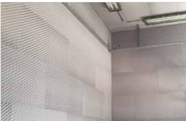
Acoustic reclamation of technical room wall partitions
