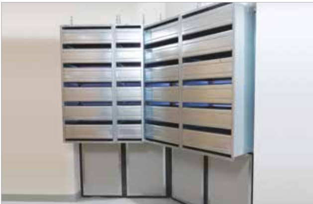
Acoustic reclamation of doors in hydroelectric power plants through the application of silencers with baffles
