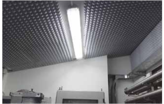
Technical room acoustic reclamation
