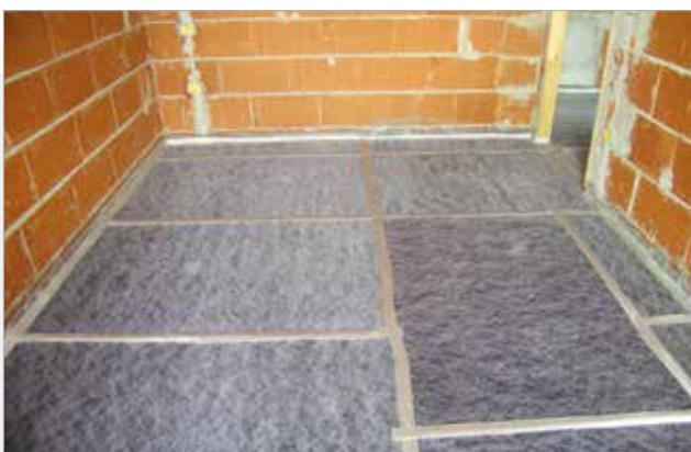
Floor acoustic insulation
