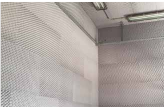
Acoustic reclamation of technical room wall partitions
