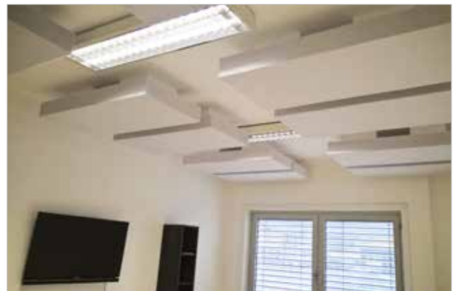
Acoustic correction inside a meeting room
