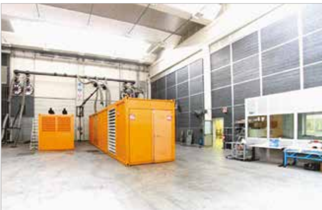
Internal insulation in a testing laboratory
