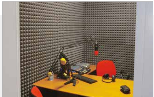
Insulation in a radio recording studio
