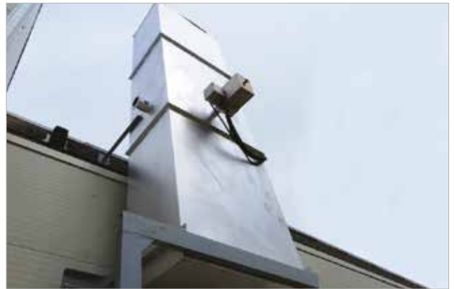
Creation of a soundproofed ducting chimney
